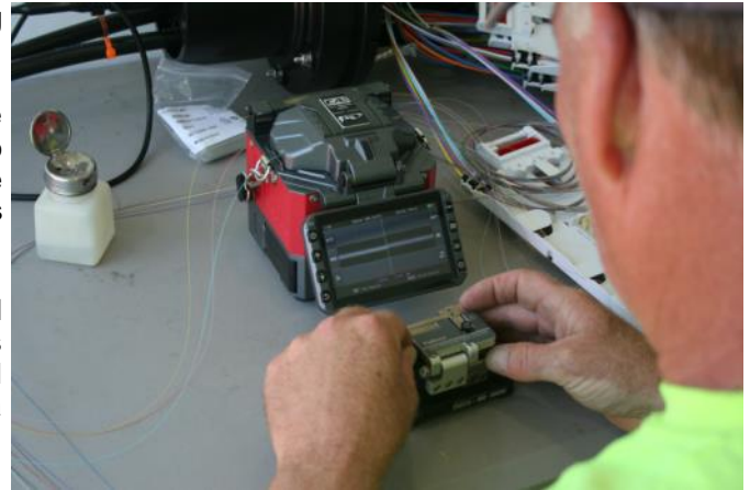
REMC's contractor splices tiny optical fibers to enable the SmartGrid Ring to communicate with all of the cooperative's substations.
